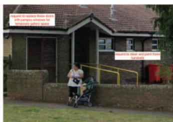
Request for permission to transform the bin store into a gallery. Image by Sam Evans
