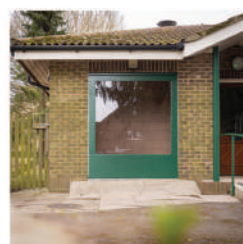
West Green Window Gallery in progress
