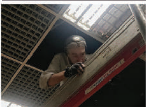
Stuart Heyes installing Unit 79/80. Image by Alex Anzenberger
