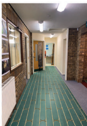
West Green Studios new floor mid installation
